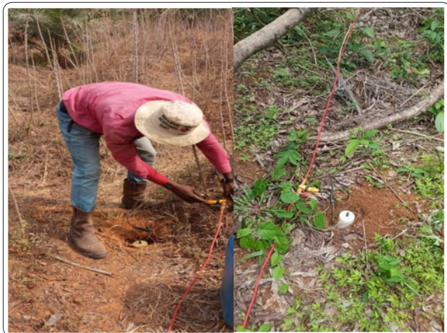
Figure 4: Electrode and porous pot installation in progress. (a) shows the connection, while (b) shows already installed Electrode and porous pot connected to 2D cable.
